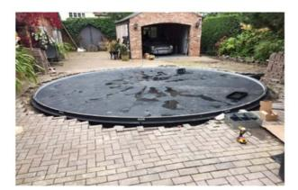
Step 6 - Block fitting within the turntable recess and cutting in to outer perimeter
