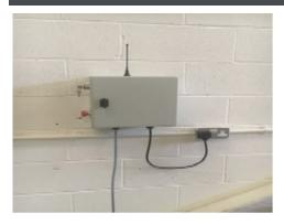
Position control cabinet within the vicinity of the turntable. Single phase 240v 13 amp supply. For outdoor use a waterproof outdoor socket or spur will be required. Route for the power cable from the control cabinet to motor unit to be given
